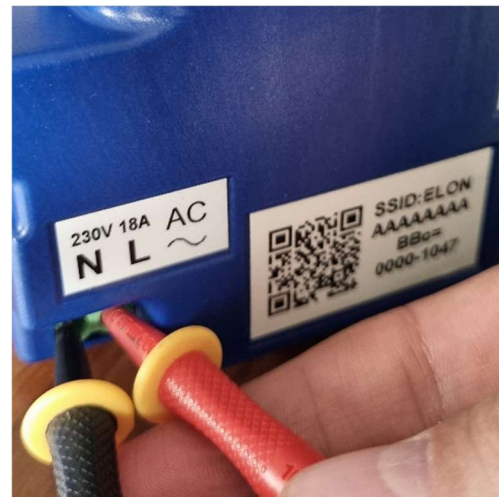
Figure A2 Checking AC voltage
