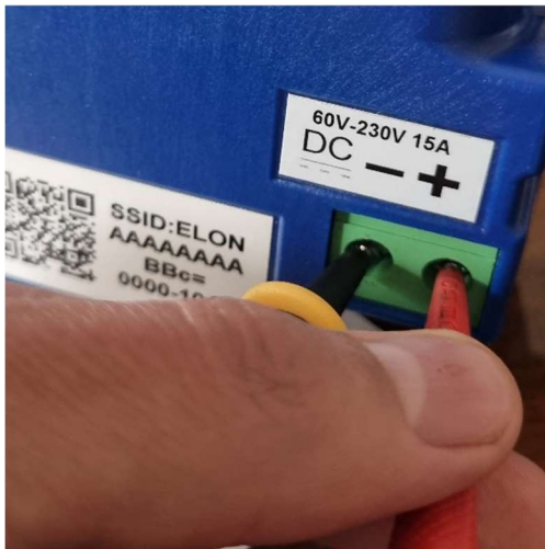
Figure A1 Checking DC voltage
